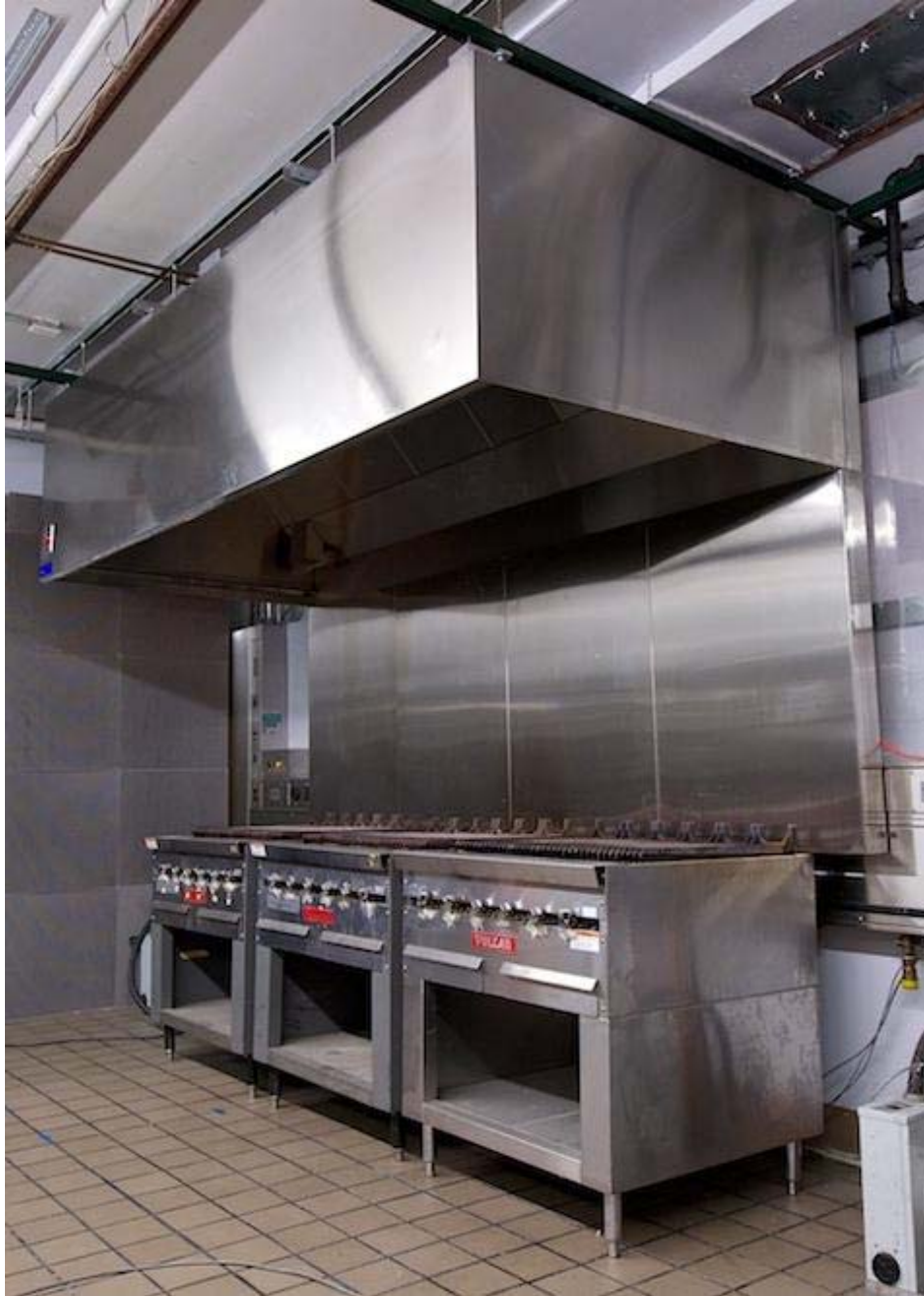
Figure 1. Streivor Wall-Mounted Canopy Hood with Integrated Backwall
