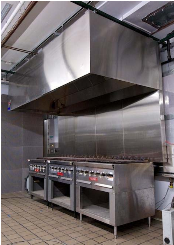
Figure 8. Heavy-Duty Underfired Gas Broiler Line
