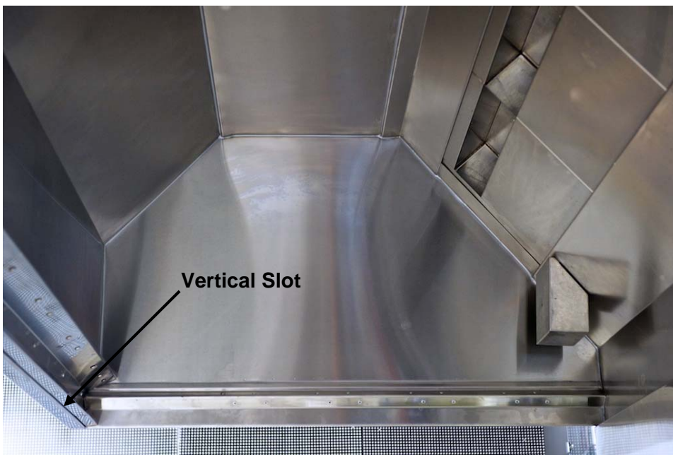
Figure 3. Interior Side Profile of Hood Showing Vertical Slot
