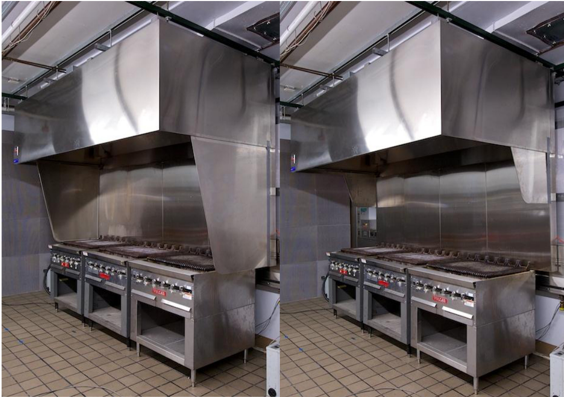
Figure 5. Streivor Hood with 40-in. by 38-in. and 21-in. by 18-in. Side Panels Installed
