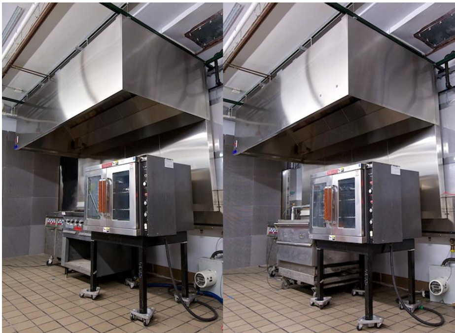
Figure 11. Fryer/Broiler or Griddle/Convection Oven Appliance Line
