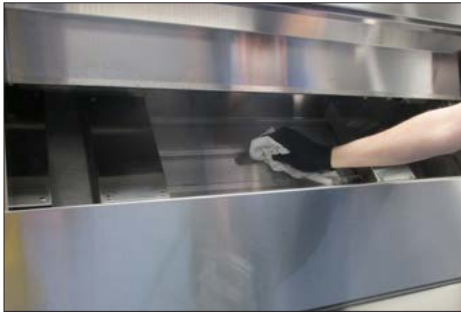
Figure 17: Cleaning UVC Lamps Located Inside Hood Exhaust Plenum
