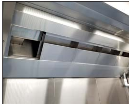
Figure 9: Install Middle Grease Extractor(s)
