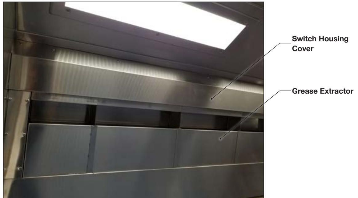
Figure 1: Extractor Positioning Switch Housing Cover
