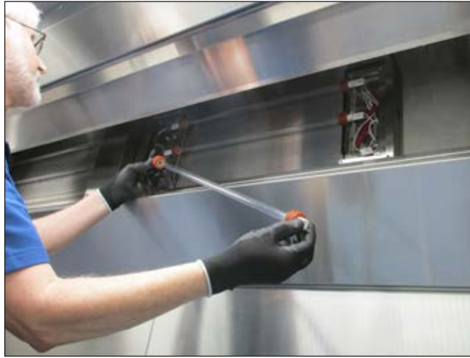
Figure 21: Removing UVC Lamp from UV Lamp Fixture
