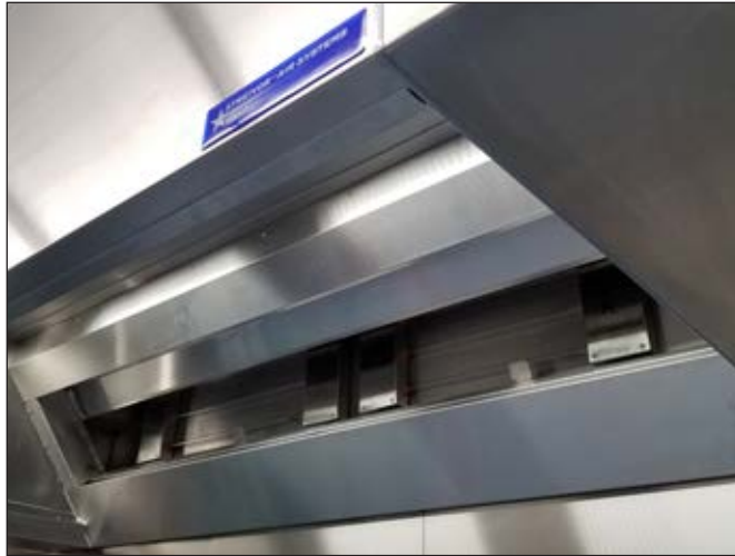
Figure 19: UVC Lamps and Fixtures Located Inside Hood Exhaust Plenum
