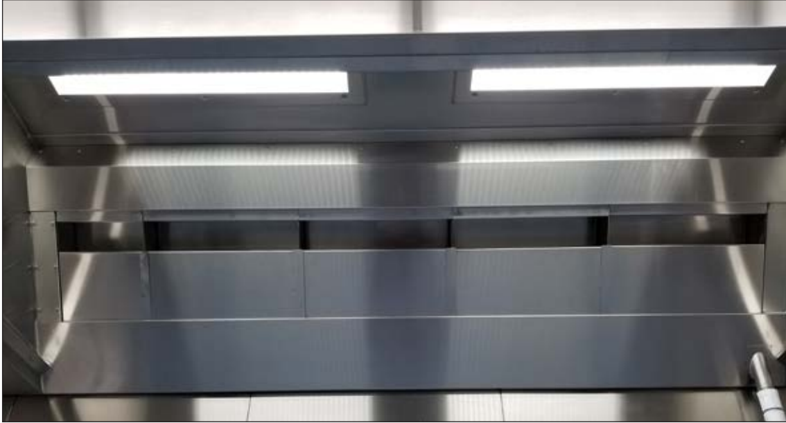
Figure 11: All Grease Extractors Installed
