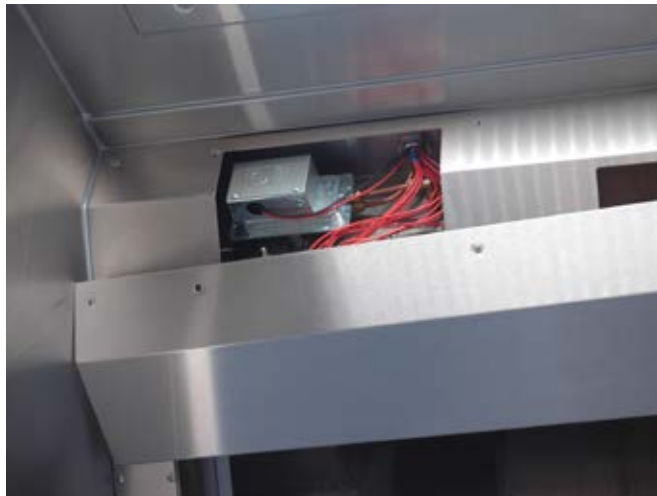
Figure 13: Pressure Switch Located Behind Switch Housing Cover
