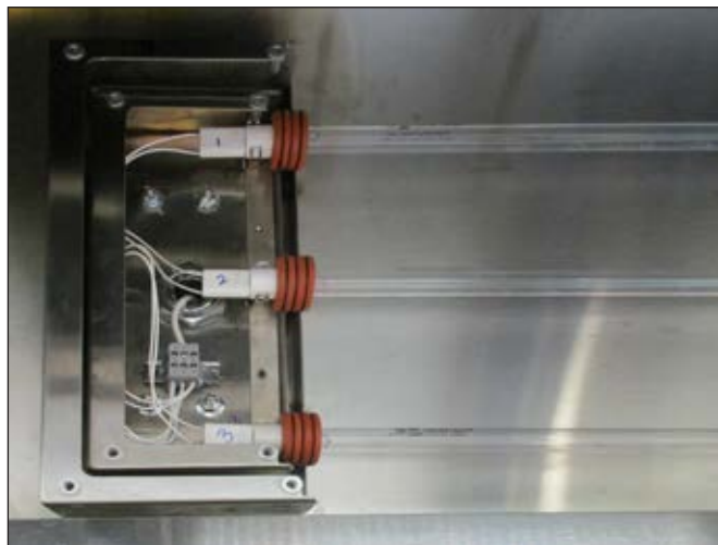
Figure 20: UV Lamp Fixtures with Cover Removed
