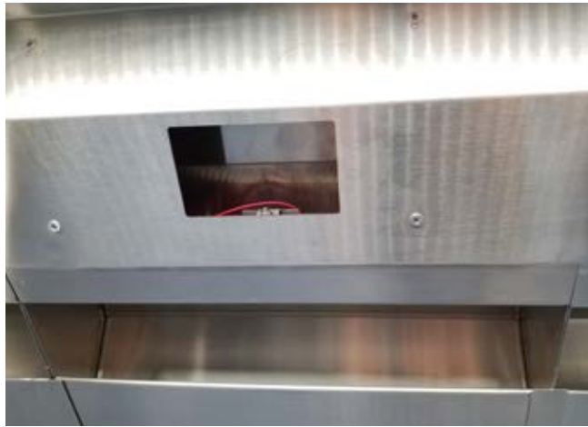
Figure 2: Extractor Positioning Switch Access Opening with Switch Housing Cover Removed
