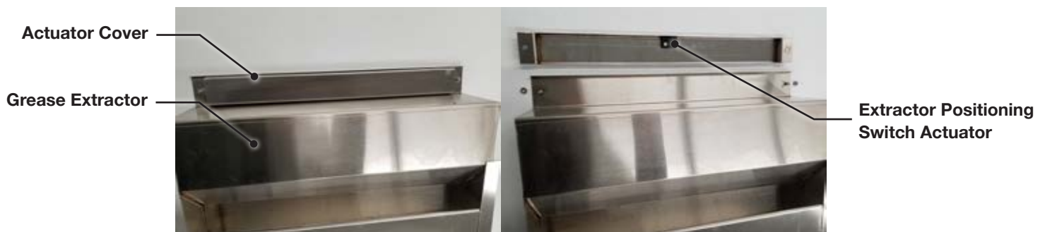
Figure 4: Extractor Positioning Switch Actuator
