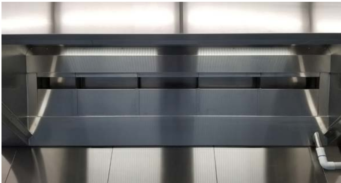
Figure12: All Grease Extractors Installed
