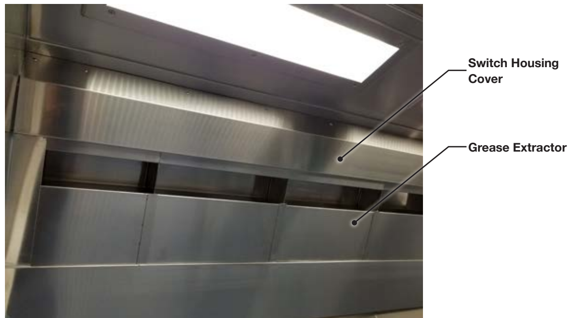
Figure 1: Extractor Positioning Switch Housing Cover
