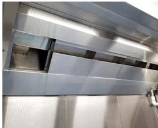
Figure 9: Install Middle Grease Extractor(s)
