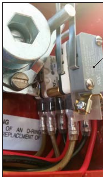
FIGURE 8B: FSS Switch for Building Alarm Circuit
