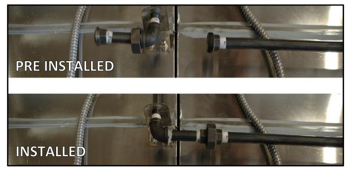
Pipe connections will be factory aligned between two hoods so they will easily rotate to face each other in order to connect the union coupling.
