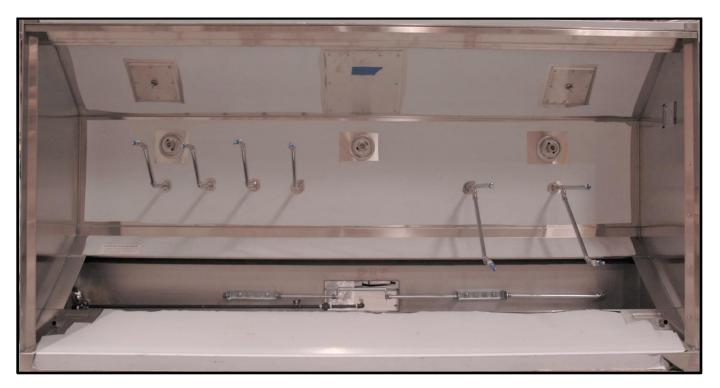
Appliance protection nozzles with swivels that do not extend below the hood canopy will be installed at the factory. Detection brackets and conduit will be factory installed in hood exhaust plenum.
