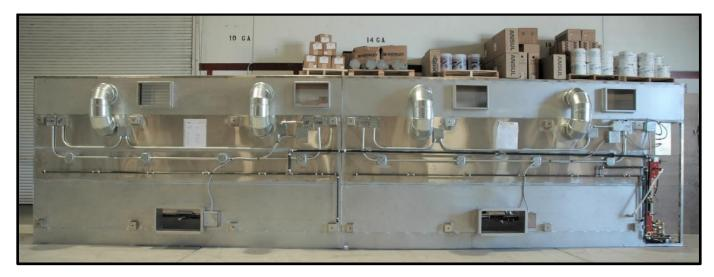
All Schedule 40 black iron pipe above hood will be completed at factory with hood interconnections and connections to system controls and tanks when hood mounted cabinets is utilized.
