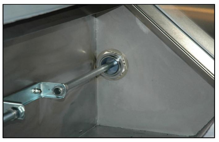
Side by side hoods sharing a common detection line are fabricated with an opening on the adjoining sides that allows the detection line to pass straight through a UL Listed quickseal which eliminates the need for corner pulley installation above the hood.
