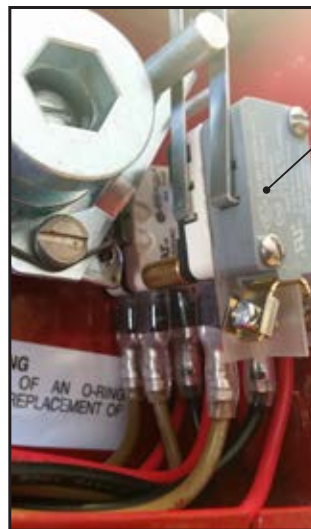
FIGURE 8B: FSS Switch for Building Alarm Circuit
