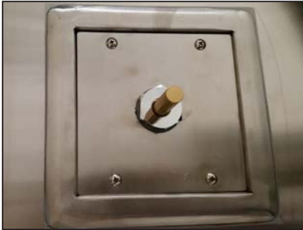
Figure 12A: Temperature Monitor Access Enclosure* (Hood Canopy Mounted Temperature Monitor Shown)
